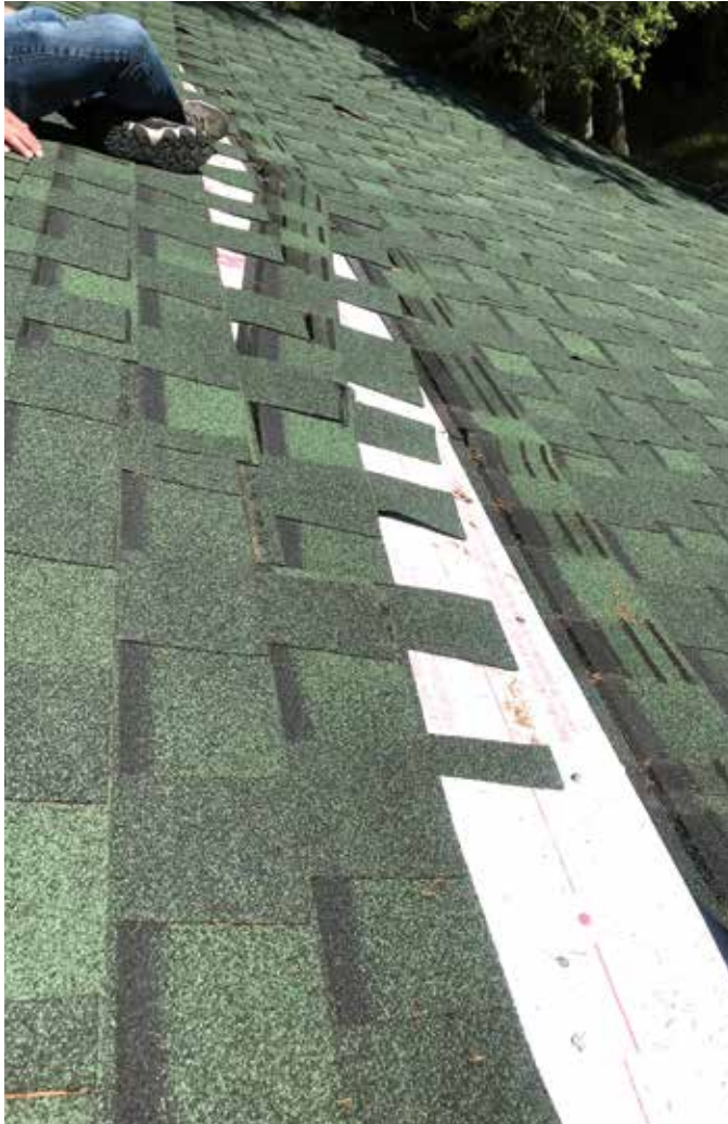
Rows of roof shingles sliding off our roof-no nails! Photo by Paul Coleman
